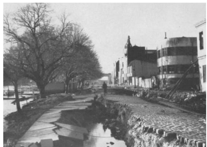
Figure 1: Ground failure along the Valdivia embarcadero from the 1960 Earthquake (Duke and Leeds, 1963)
