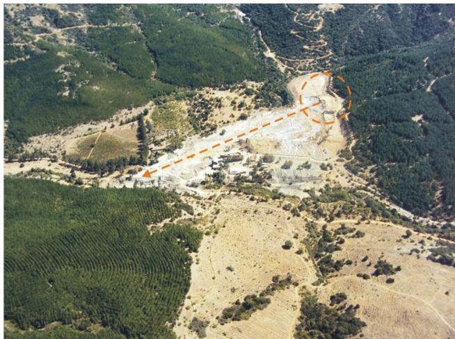
Figure 2: Las Palmas tailings dam after the collapse generated by the 27 February 2010 earthquake (Villavicencio et al. , 2014)
