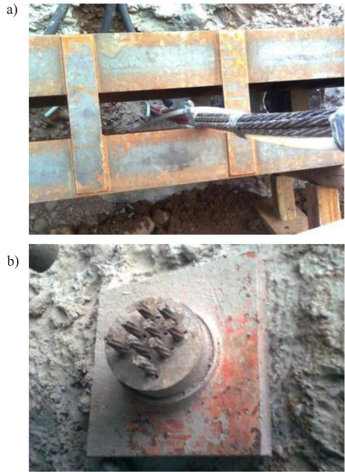
Figure 7: Detail of anchor head; a) Energy Anchor and b) standard anchor
