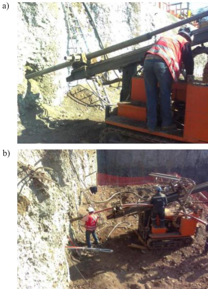
Figure 6: Installation of Energy Anchors: a) ground drilling, and b) cable and HDPE pipes are inserted.
