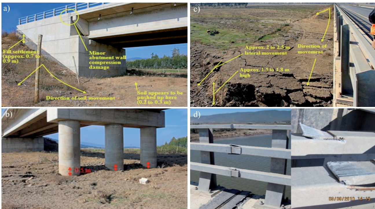
Figure 1: a) North abutment, b) lateral displacement towards the river, c) soil settlement at interior pier at northeast abutment (FHWA, 2011), and (d) handrail failures at the bridge deck
