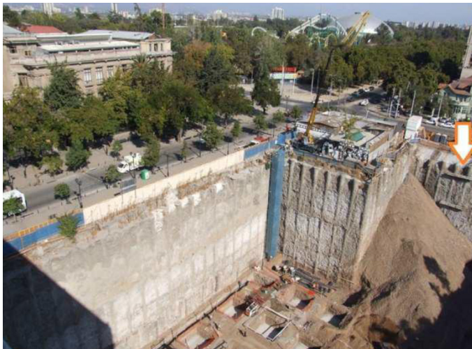
Figure 3: View of vertical excavation and instrumented energy piles (indicated by an arrow)
