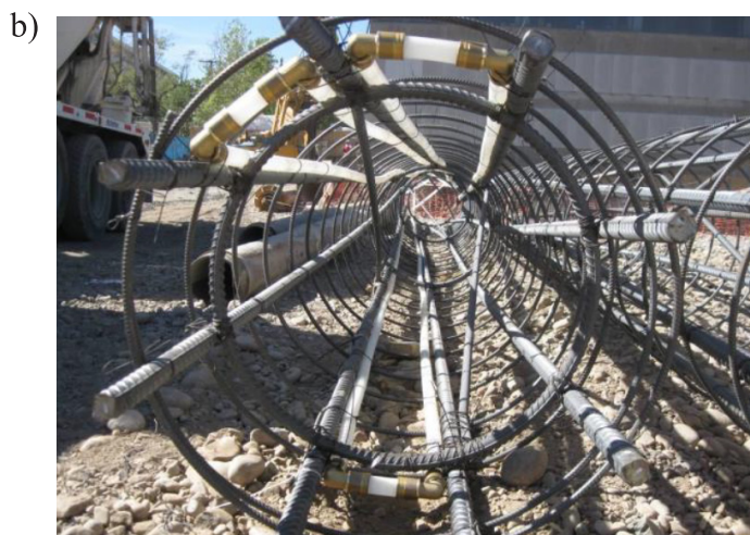
Figure 4: (a) Configuration of HDPE pipes in the energy piles and (b) energy pile being assembled on the field
